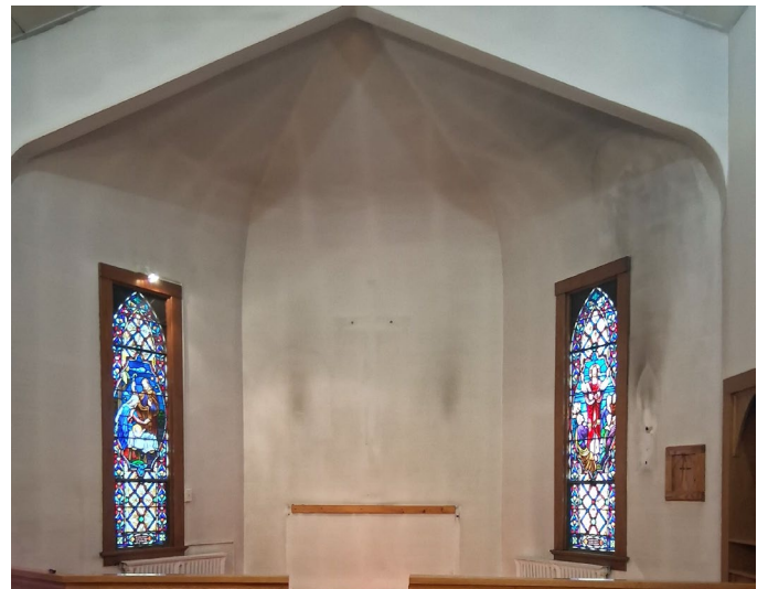
Our Sanctuary prior to cleaning, repairs and painting
