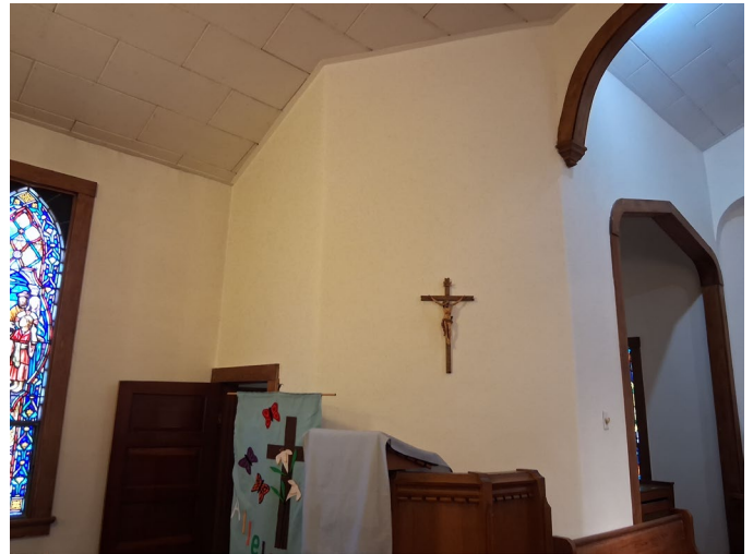
After cleaning, repairs and painting
