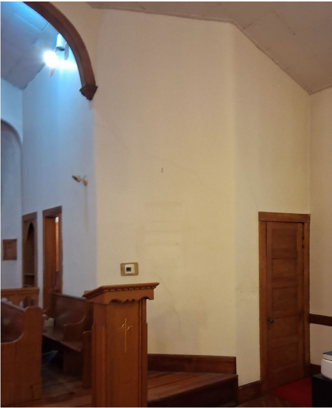
Prior to cleaning, repairing and re-painting
