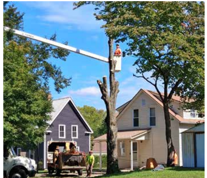
Tree being removed
